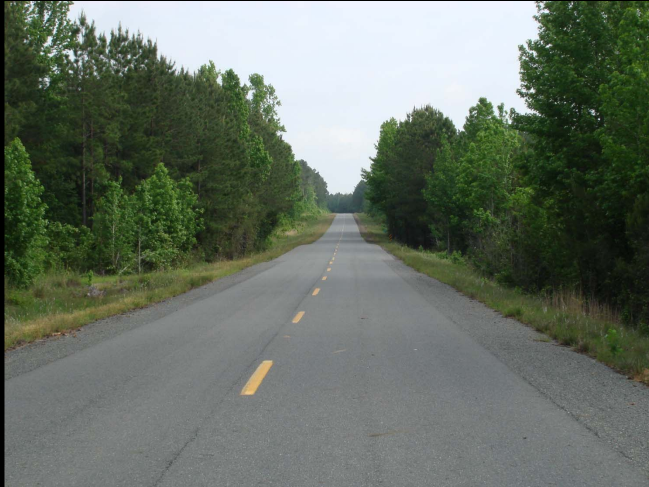
LA 464 (Vernon Parish) – 1999 with “Hot” RAP Shoulders Tie-In to Adjacent Project (2001) with “Plain” RAP Shoulders
